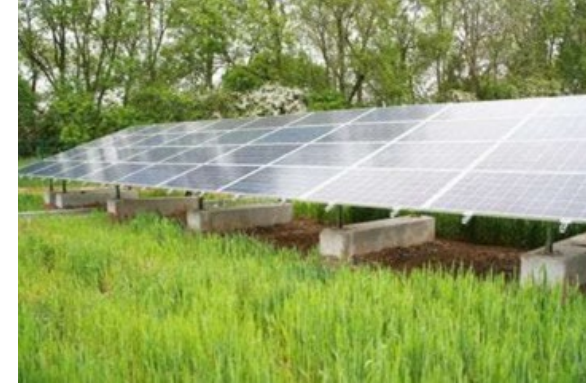
Panels with Concrete Feet
